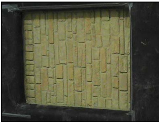
Concrete Panel in Test Wall
